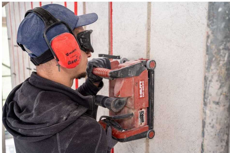
Fig. 16 Milling in the pipes into the concrete blocks @Sozialbau AG
