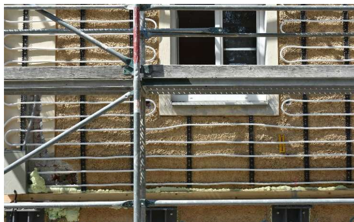
Fig. 12 Project 'Wohnen findet Stadt' Fixing the pipes to the existing masonry @ FH Salzburg
