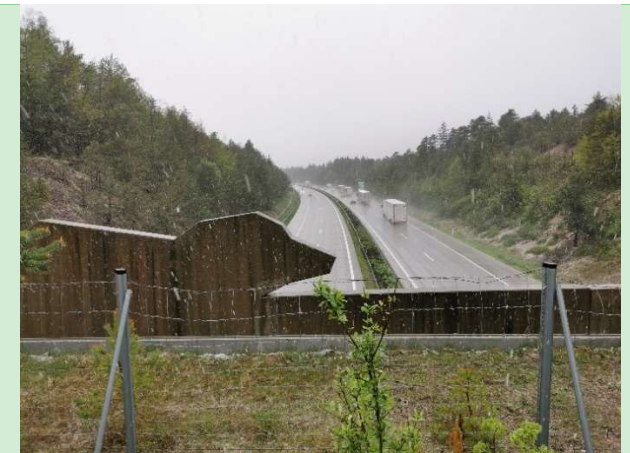
Figure 16: Wildlife bridge across the highway A2
