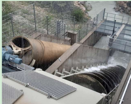
Figure 15: Fish lift at river Gail.
