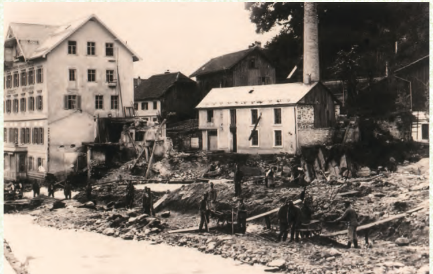
Cleaning up after the disaster, 1910. Source: © Wirtschaftsarchiv Vorarlberg.
