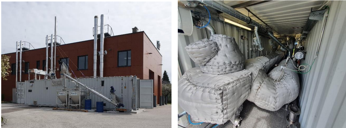
Figure 8: left: Pilot Scale pyrolysis plant from outside; right: pyrolysis plant inside container, pyrolysis reactor on left and gas burner on right side
